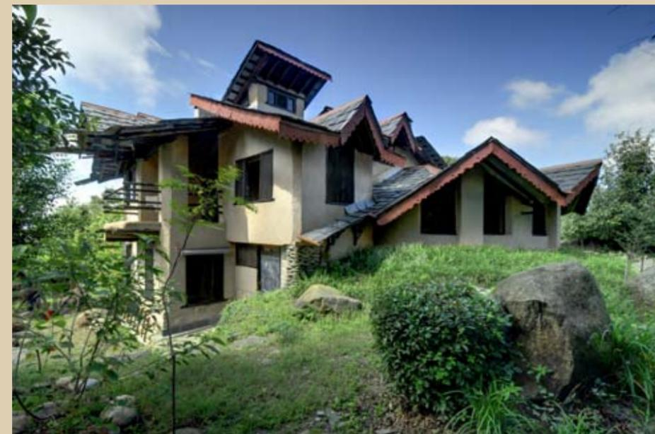
*Above: Walls are constructed out of Adobe (sun dried mud bricks of size 6x12x3 inches) created at site from earth harvested during excavation. Wall thickness is generally 18 inch wide and the wall is plastered in mud that has organic fiber additives to ensure that the plaster does not crack. Pulped waste paper can also be used to provide the fiber.*
