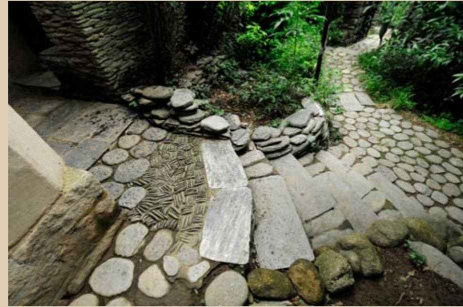
*Left: Slate, a common building material in the area is used for floors, steps and roofing. Pathways are paved with slates shaped by the near by river. Large river gravel, organized in a pattern at the entrance, forms a natural doormat.*
