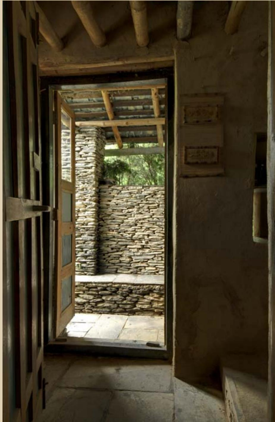
*Left: The entrance porch is created with stacked stone with a part of the wall broadened at the base to form a seat. Slate moves up one level and becomes the surface of the seat. Stacked stone masonry is one of the elements of the Himachal vernacular. Didi re-interprets it in her buildings in a designed manner.*
